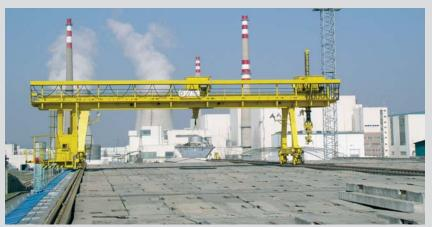
The repository consists of 112 reinforced concrete vaults arranged in four rows of 28 vaults each. The waste drums are placed within the vaults by a gantry crane; the operator's cabin is shielded to protect the operator from radiation exposure.
