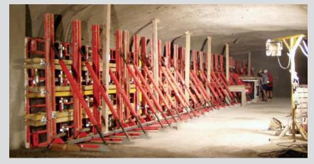
The "Realisation of Closure of Chambers at the Richard Repository" project; the construction of the inner wall of the hydraulic cage.
