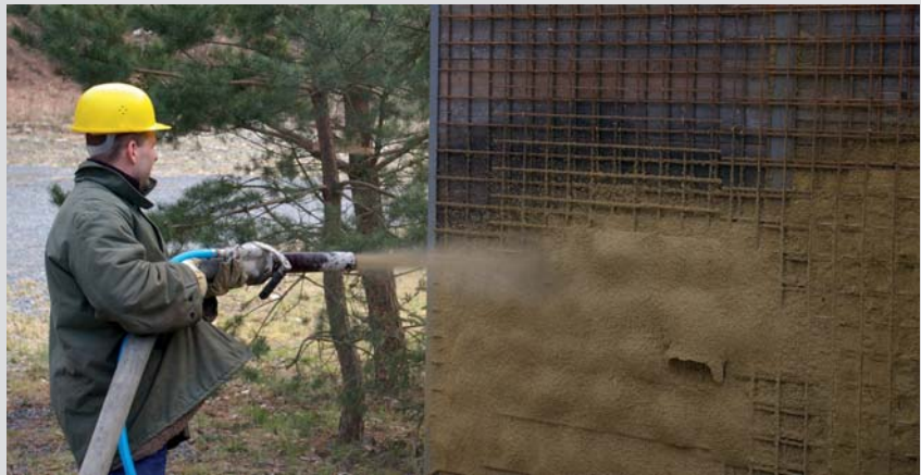
Experimental research of shotcrete backfill technology. (Centre for Experimental Geotechnics, Czech Technical University). Shotcrete backfilling on the experimental wall at the Josef facility.
