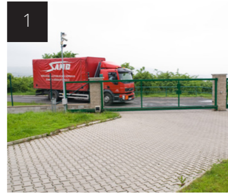
1 A truck with radioactive waste enters the Richard repository complex
