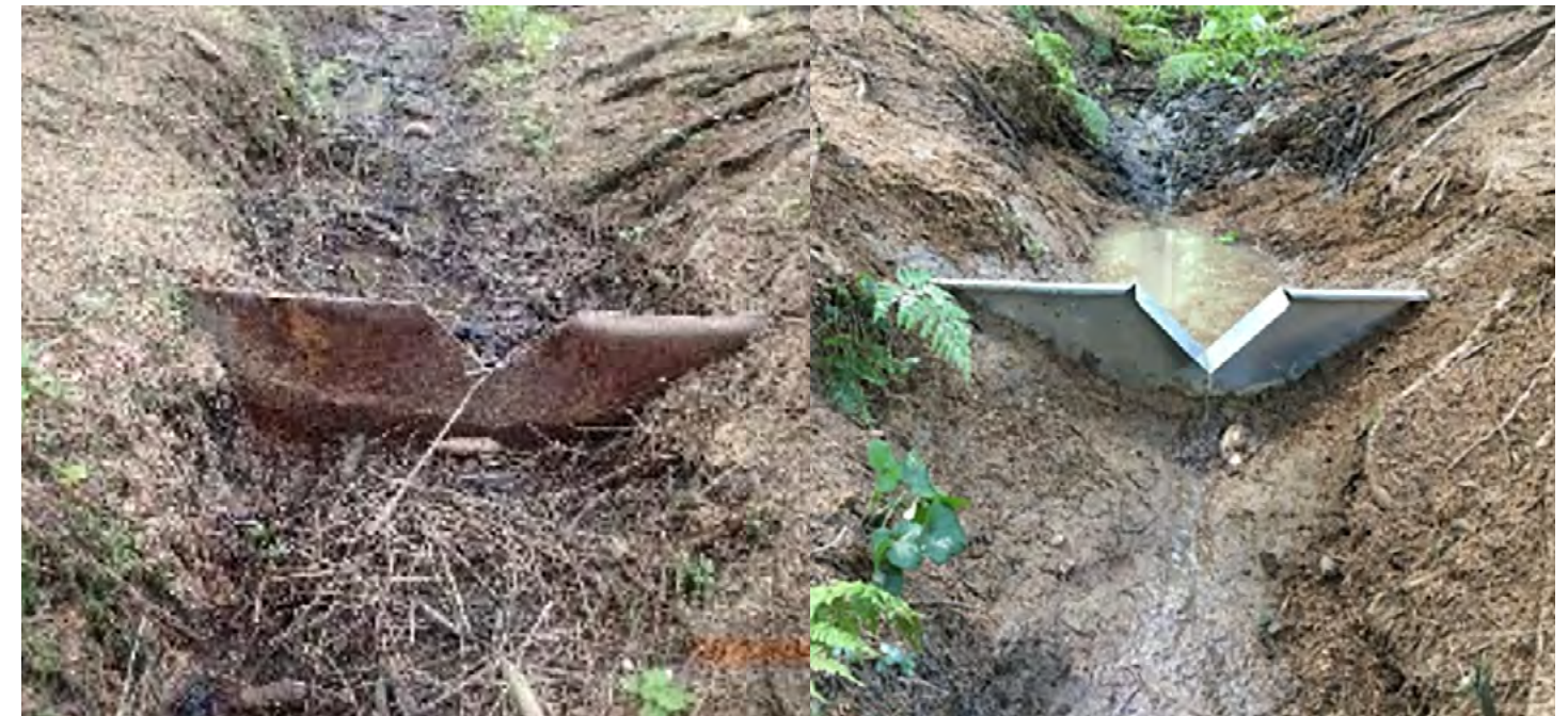
↑ Original and new water collection points on the surface of the site
