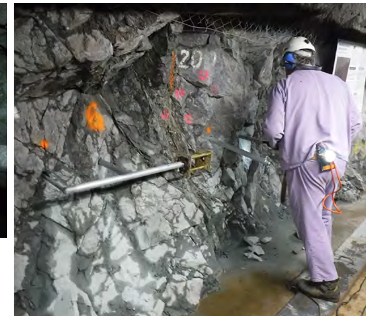
↑ Installation of extensometer mounting brackets in the BZ-XIIJ crosscut
