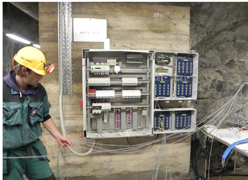
← Installation of a junction box and cabling
