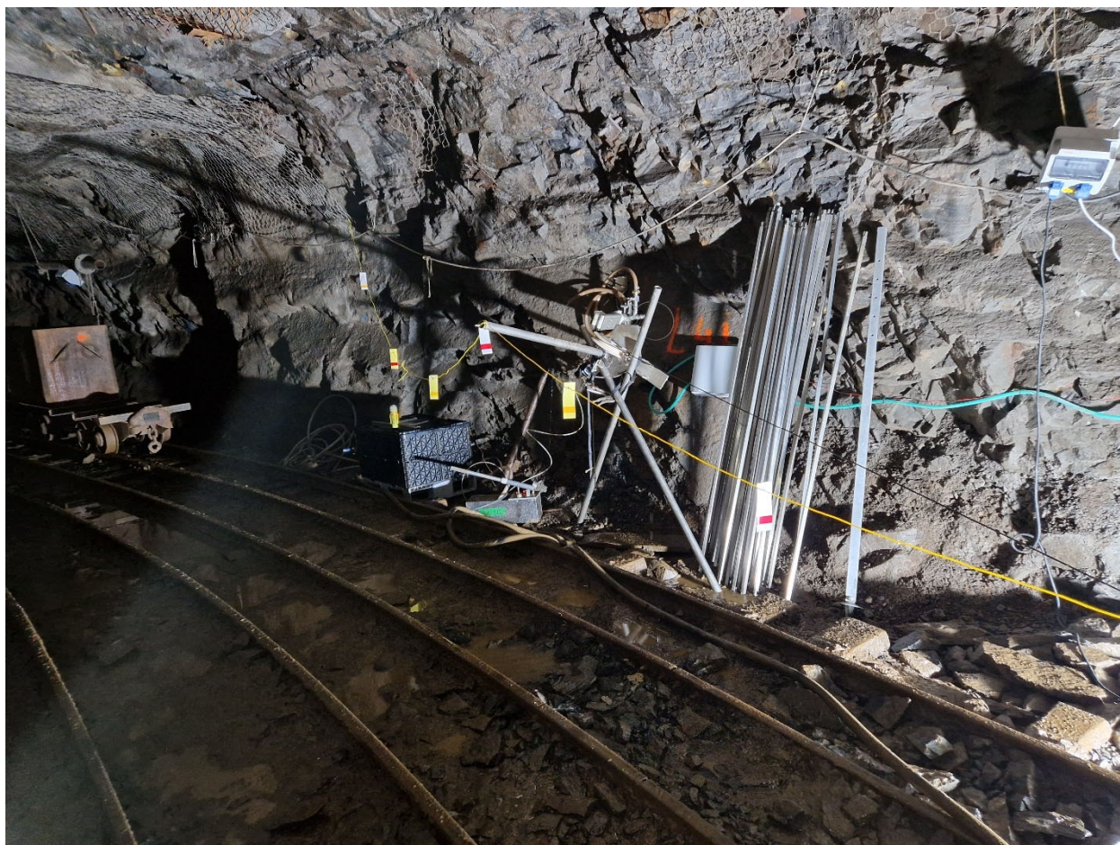
Figure 2. Borehole S-33 commenced at the tunnel wall.
