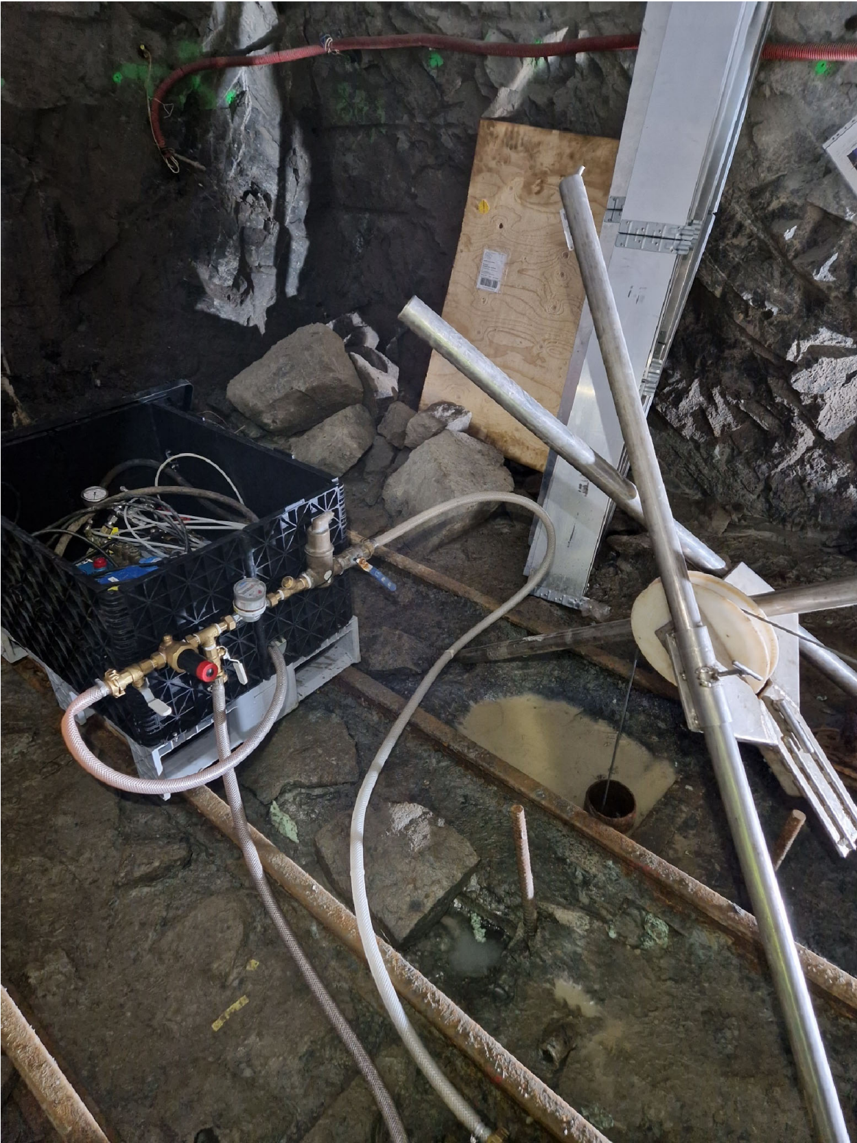
Figure 3. Borehole L7-87D commenced from the tunnel floor.
